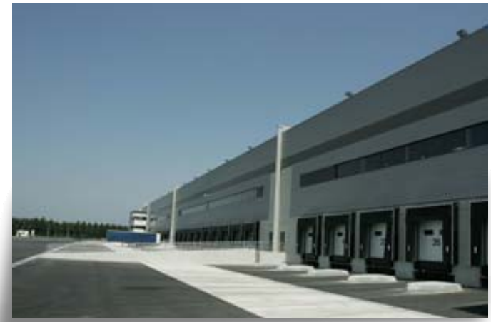
Loading cells at the Cestas warehouse
